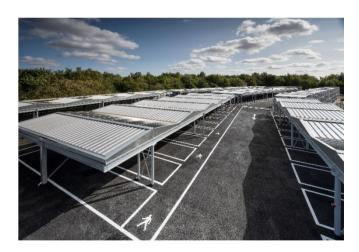
On the top deck we installed 276 solar panels which provides power for the EV charging and a canopy to cover cars parked on the top deck. The solar generated is supplied back to two inverters installed during the works in a
