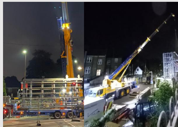
Lift shaft installation at Isleworth Station
