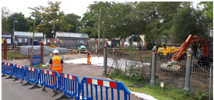
Works in progress
