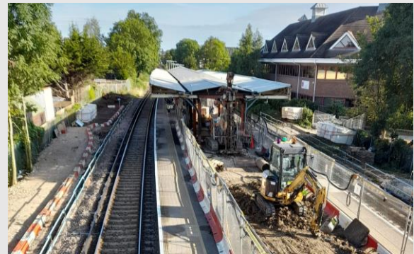
Works at Motspur Park
