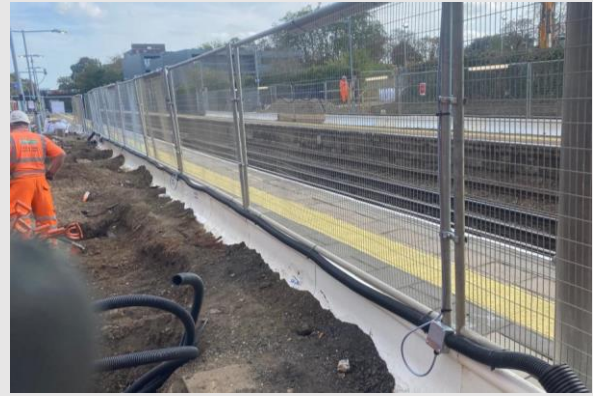
Works at Barnes Station
