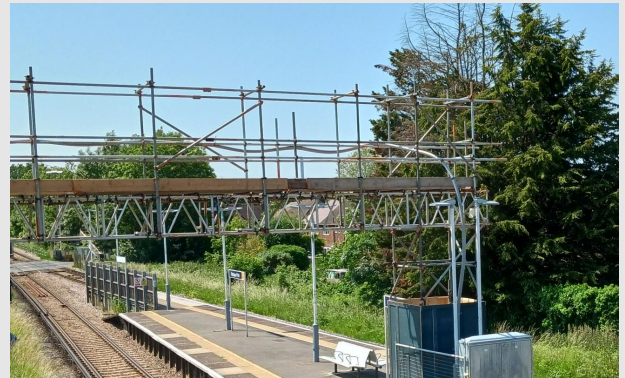
Construction of service cable bridge at Motspur Park.
