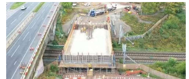
Figure 2 – Bridge construction over the Great Western Railway
