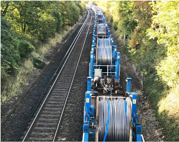
Figure 2 – HV Feeder Renewal
