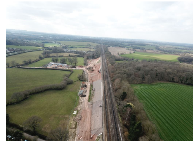
Figure 1 - Ashmead Embankment Drone Image
