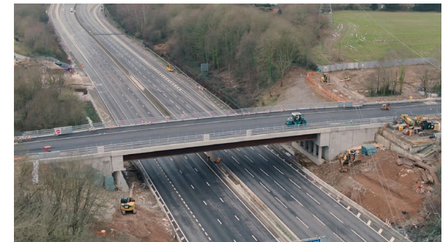
Figure 1 - Bridge in place
