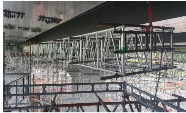
Figure 1 - Rolling Deck Launch
