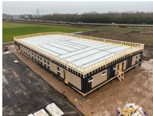
Figure 3 – SIP's erection
