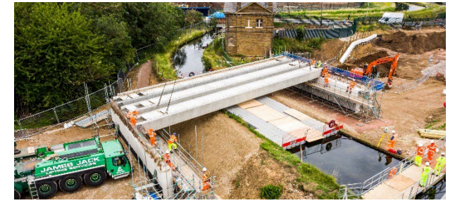
Figure 1 - Bridge Installation over canal
