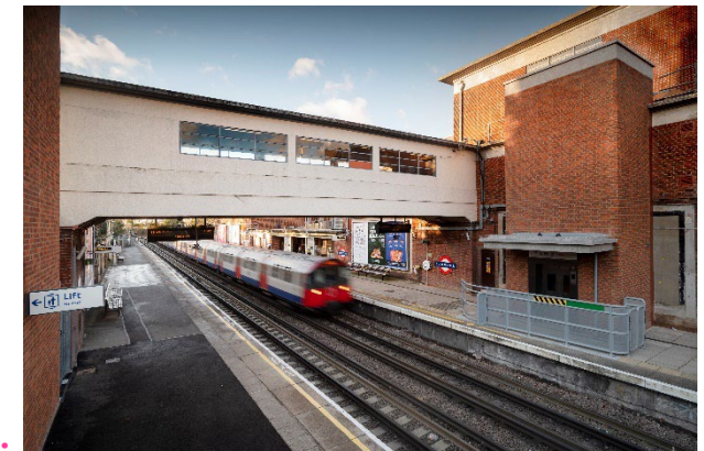
Figure 1 - Sudbury Hill Station
