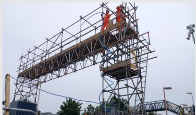
Cable bridge construction underway at Motspur Park.
